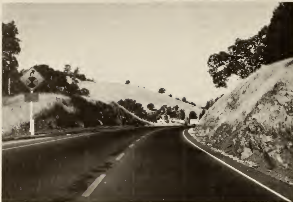
Figure 59 Primary Sign C And Supplemental Message (Amador Central Crossing)
